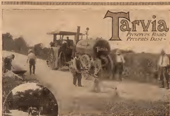
The illustration shows "Tarvia X" being applied under pressure on the wearing course—at this step the road is about half constructed. The view in the circle is the finished road. Note that the speeding auto leaves no trail of dust.
